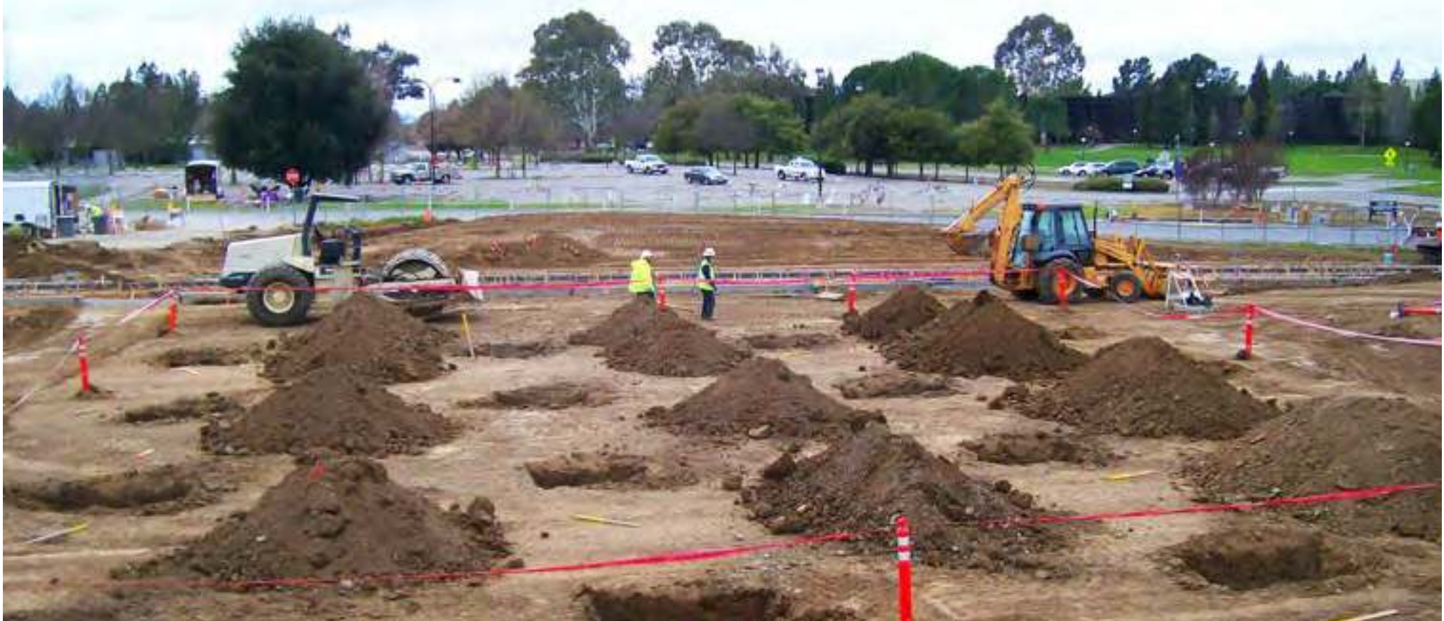
Cutting & filling of earth on a job site during rough grading
