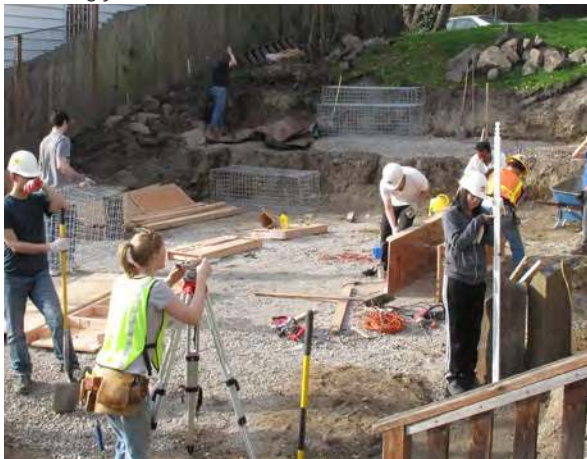
Checking final elevations
