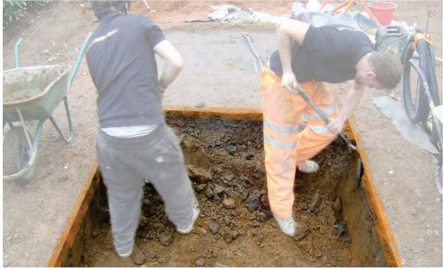
Manual excavation to establish a reflecting pond
